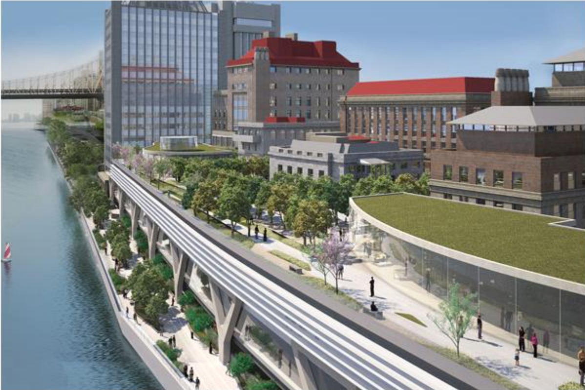
Turner Construction is the muscle behind the renovation of Rockefeller University on the Upper East Side.
